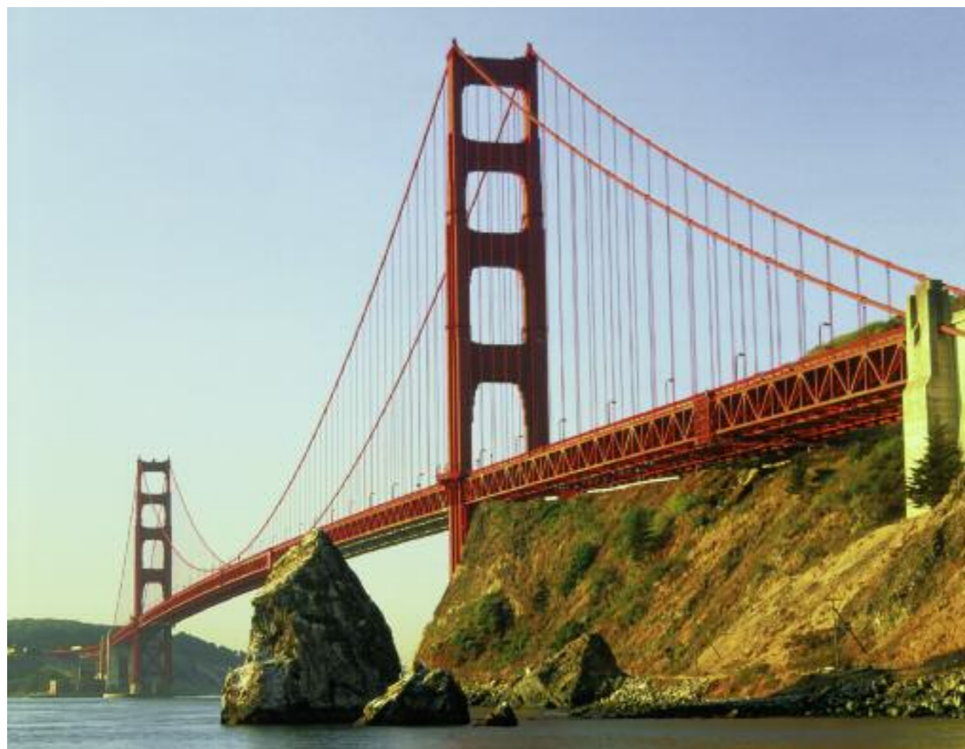
Golden Gate Bridge, San Francisco
